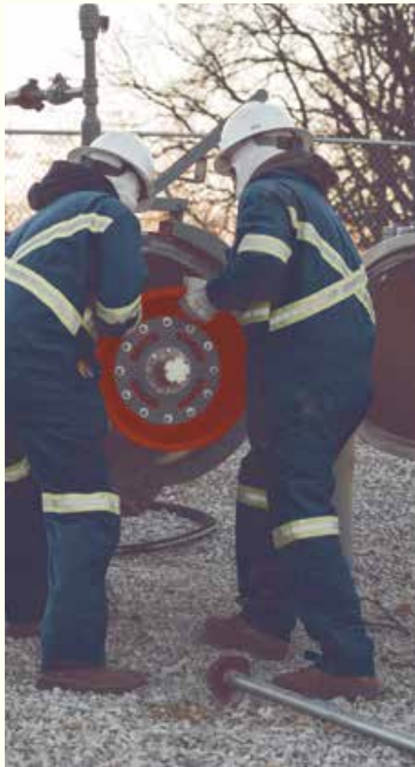
Employees near Sapulpa, Okla. insert a “pig” as part of procedures to inspect a pipeline. Pigs are used to perform various maintenance tasks and inspections on certain pipelines.
