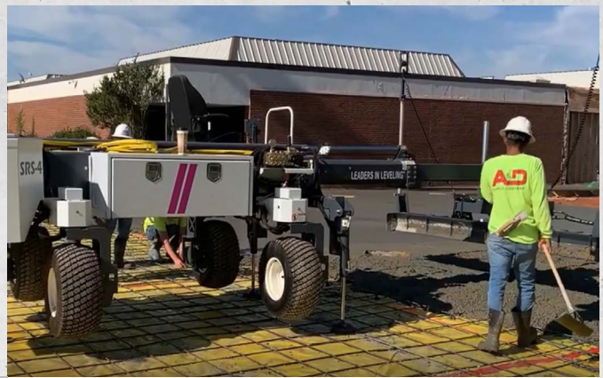
↑ SRS-4 Boom Laser Screed® in action
