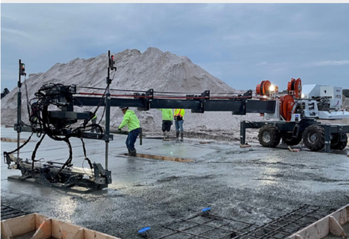
↑ S-PS50 Laser Screed® in action
