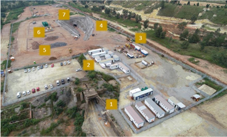
IMAGE 6: COMPLETED INFRASTRUCTURE AT QALA SHALLOWS
