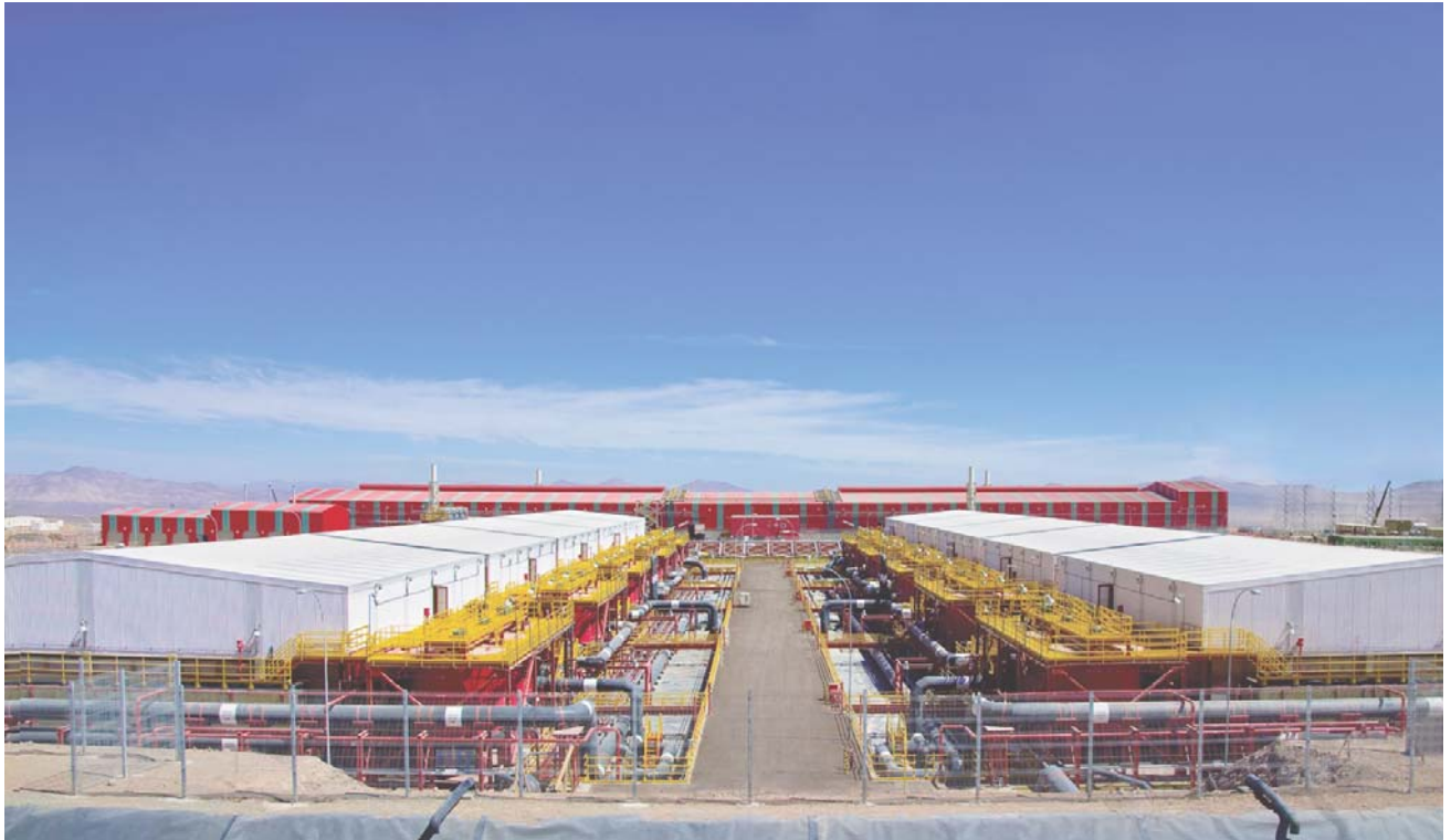
Figure 1 - Bateman Tenova designed and built Copper SX EW plant in Chile. SX units are located in two banks in foreground. Electrowinning refinery is housed in the large building at rear. Plant is similar in conceptual layout and size (1.5mtpa) to the proposed NiWest processing facility.
