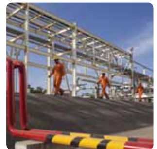
Top: Raageshwari gas terminal at Rajasthan, Cairn India.
