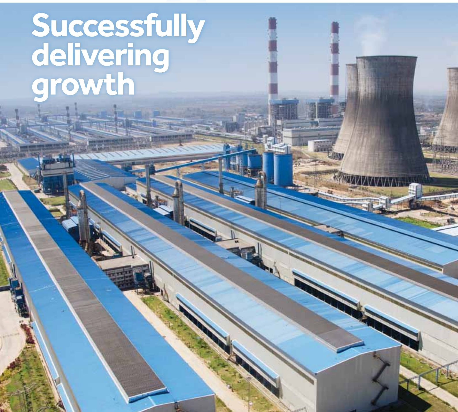
Above: Aerial view of Jharsuguda smelting complex.
