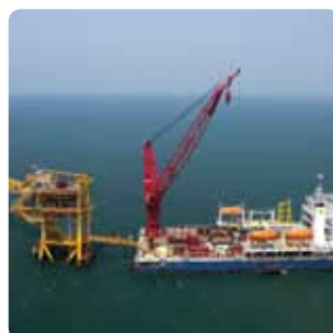
Above: Ravva offshore terminal, Cairn India.
