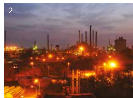
2 Night view of Chanderiya smelting complex, HZL.
