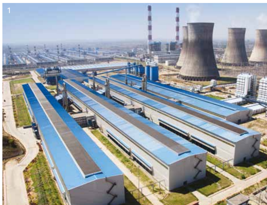
1 Aerial view of Jharsuguda smelting complex, Sesa Sterlite.
