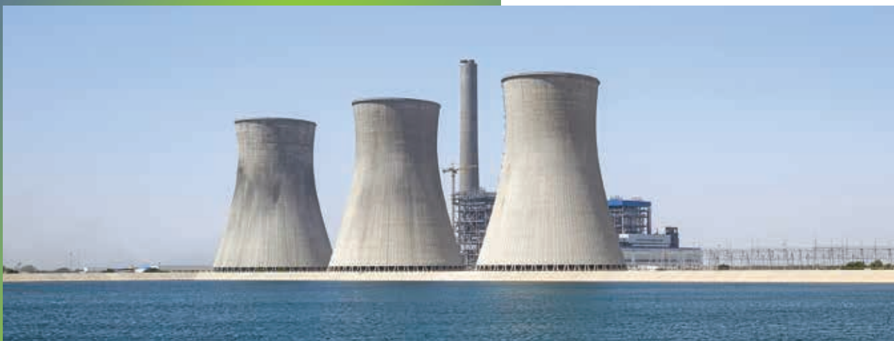
Below: Power Plant at Jharsuguda
