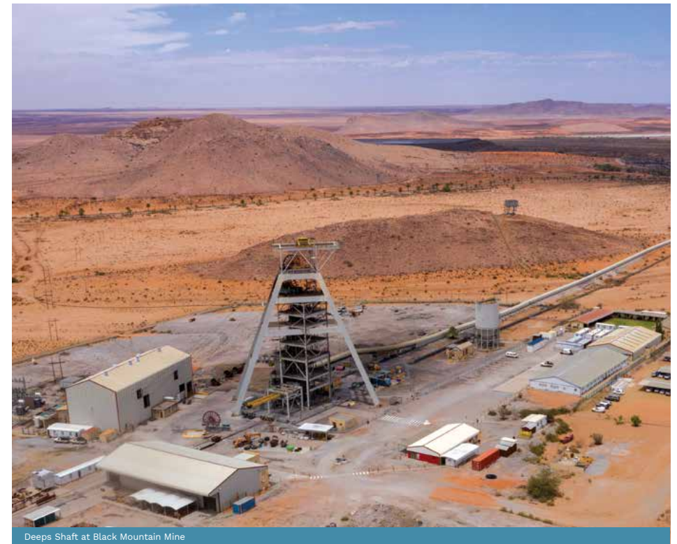
Deeps Shaft at Black Mountain Mine
