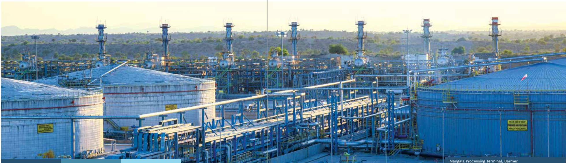
Mangala Processing Terminal, Barmer
