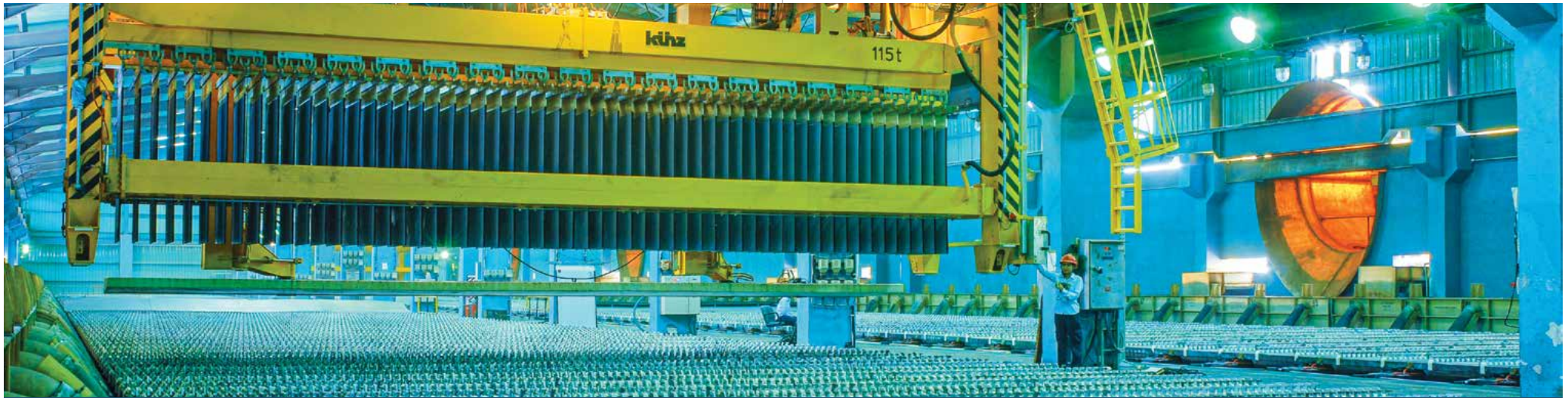
Zinc Smelter, Chanderiya, HZL
