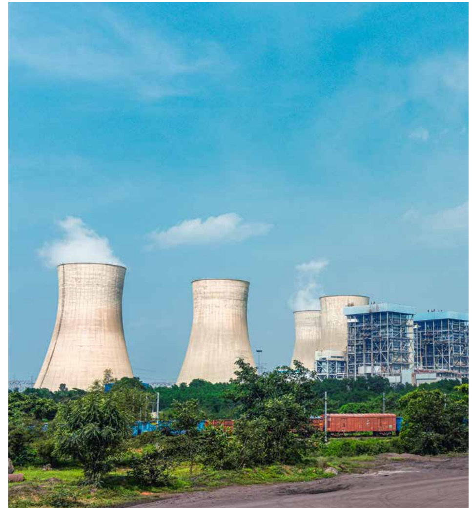
TSPL Facility, Side View
