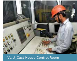
VL-J_Cast House Control Room
