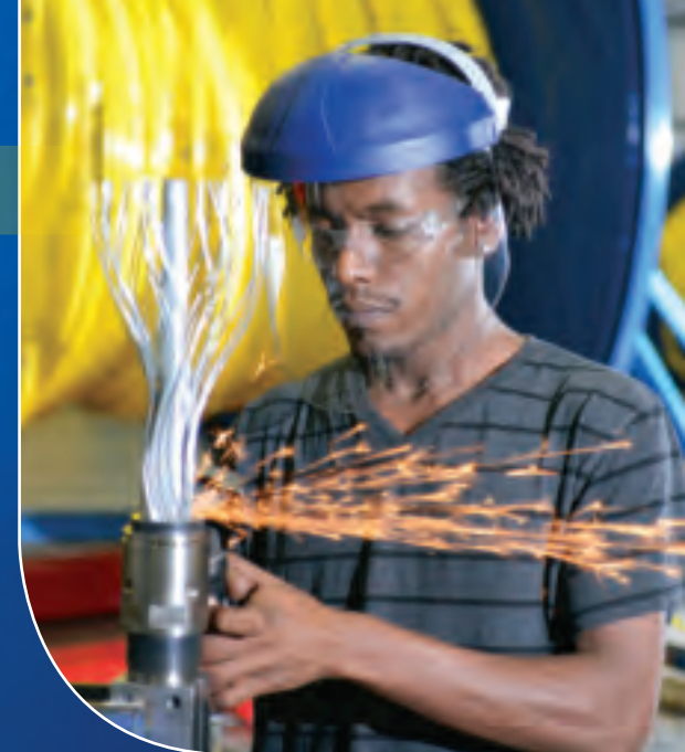
The ends of each cable section must be “terminated” and connection hardware installed.
