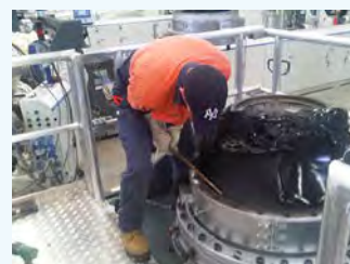
THE HEIGHT OF THE PLATFORM MEANS THAT OPERATORS CAN WORK AT THE SAME LEVEL AS THE TOOLING MACHINE.
