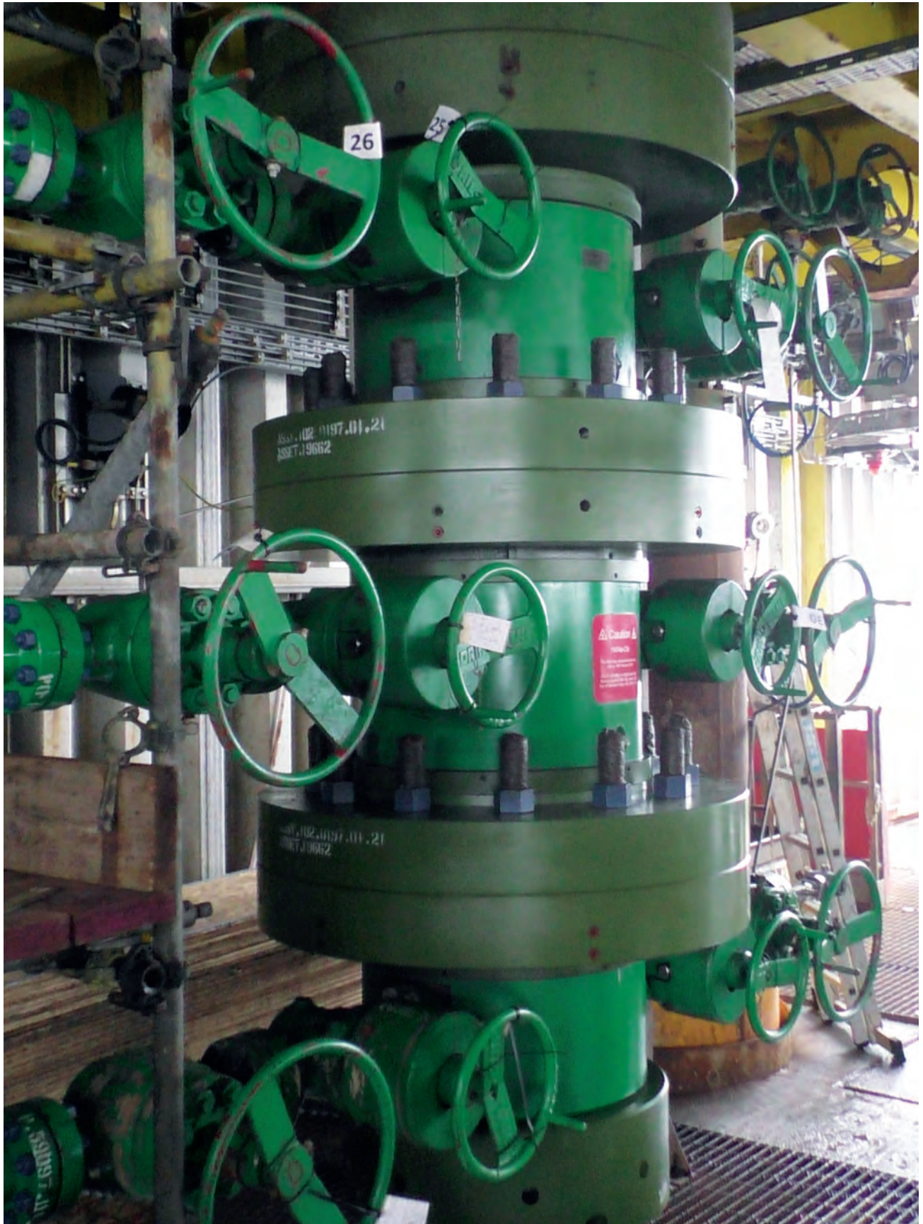
POS-GRIP "HG" Production Wellhead recently intalled offshore
