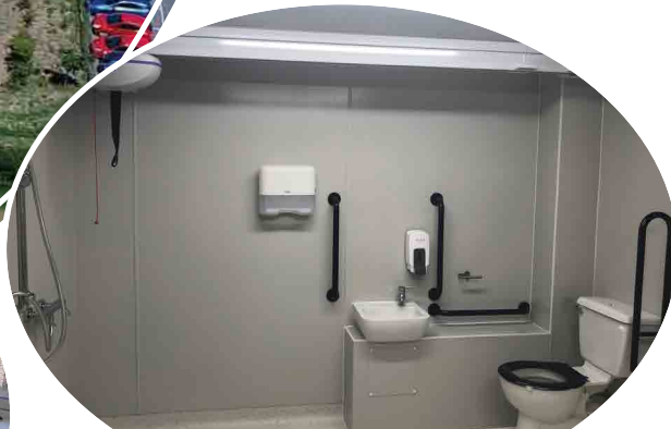
Bathroom Hoists / Tracking
