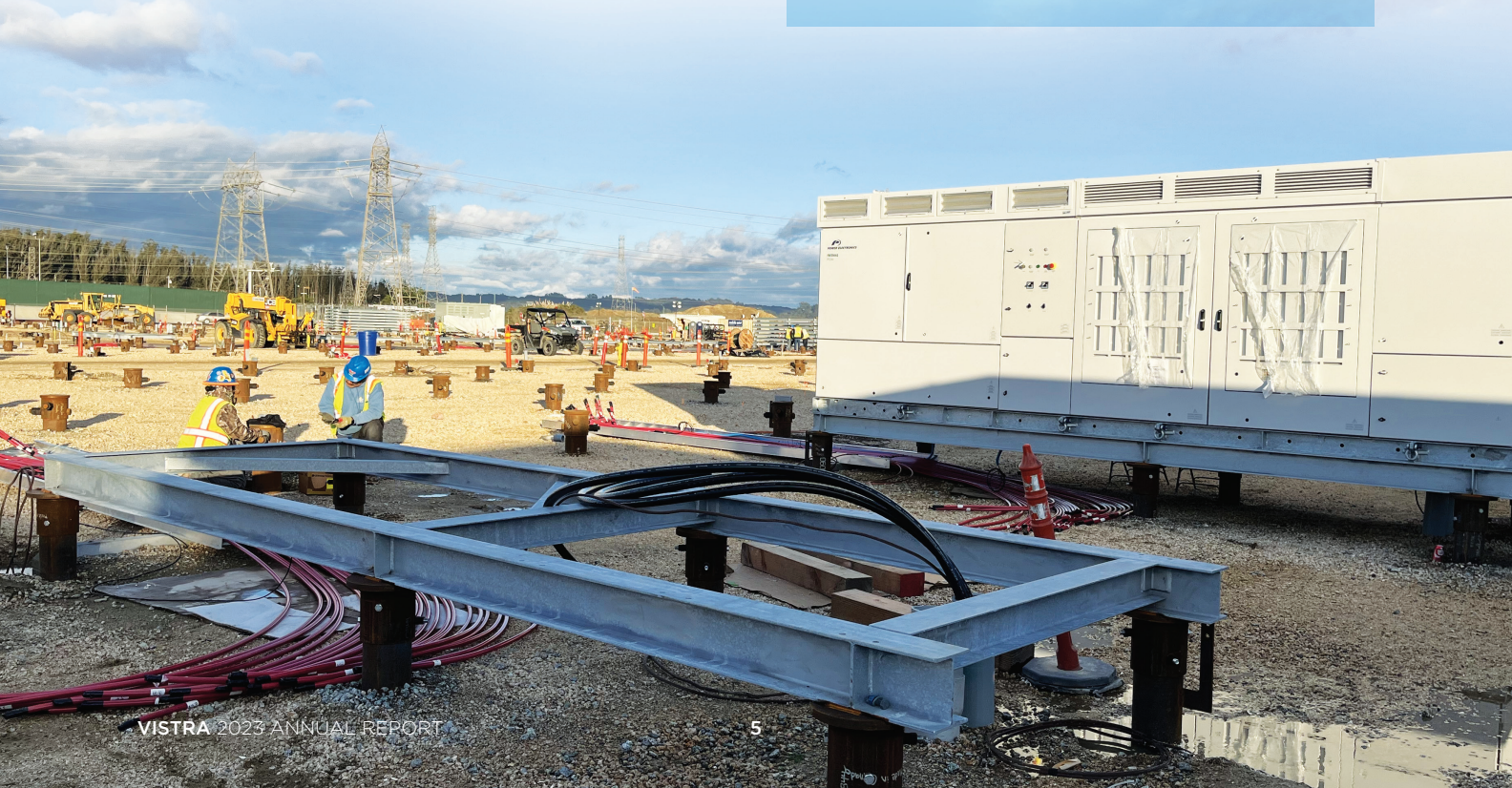
Below: The Phase III expansion of the Moss Landing Energy Storage Facility—made up of 122 individual containers that together house more than 110,000 battery modules—was completed in summer 2023 on schedule and within budget in just 16 months.
