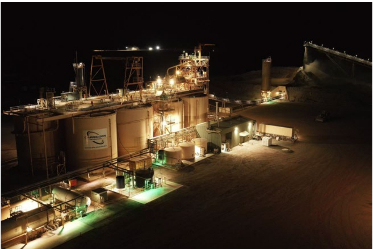
Processing plant at Karlawinda Gold Project
