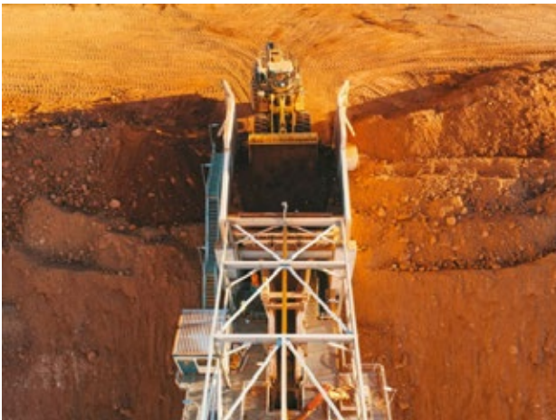
ROM Loader putting material into the crushing circuit at the Karlawinda Gold Project
