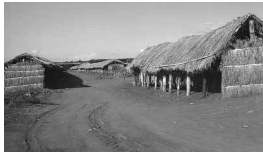
Malawi curing barns.
