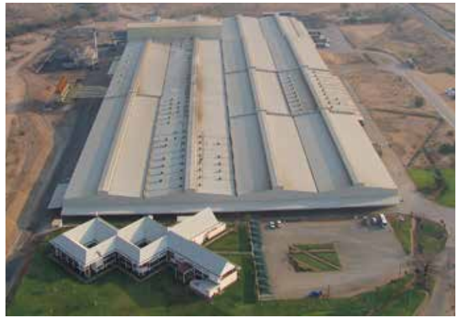
Universal processing facility in Tete, Mozambique, 2006.
