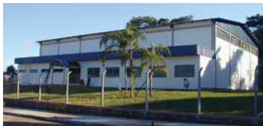
Community center built by Universal as part of the Citizen Program.
