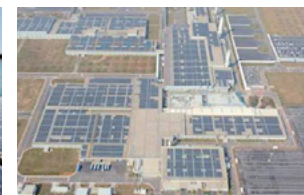
Solar panels at a new plant in China
