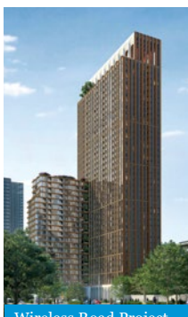
Wireless Road Project
