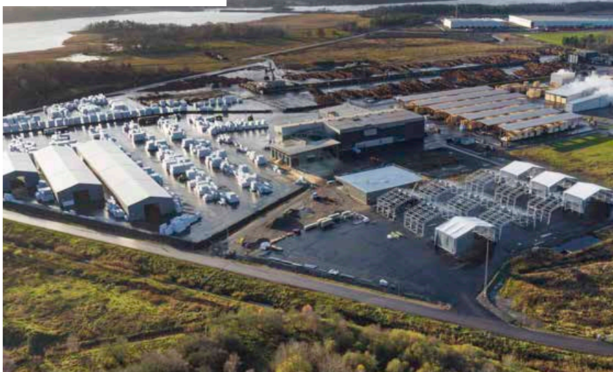
The wood treatment plant at Braviken Sawmill will be operational in 2018.
