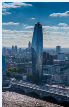
Most Considerate Site (>£50m) One Blackfriars
