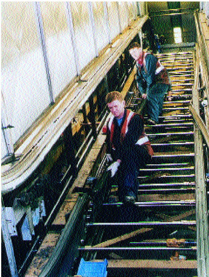
Installation of Renolube chain on one of Merseyrail's public escalators
