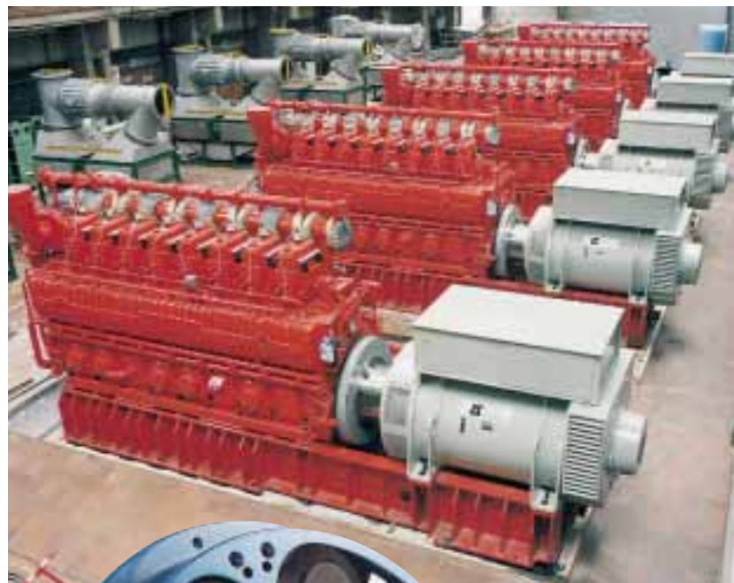
Severn Trent Water has used Renold Hi-Tech couplings to link some of the UK's largest gas engines to generators in a heat and power operation fuelled by sewage waste gases.
