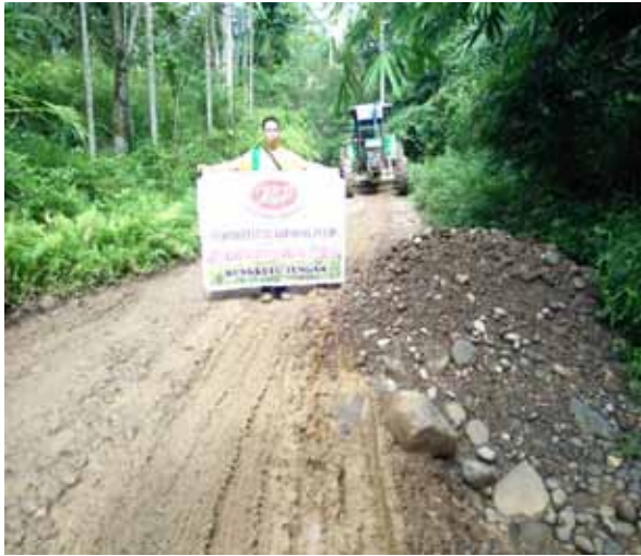
Repairing public road
