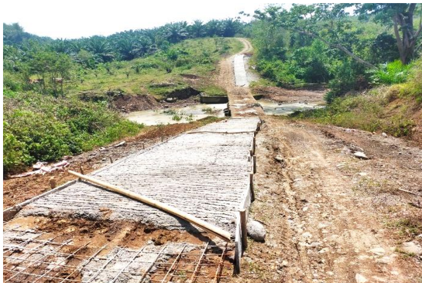
Upgrade of public roads
