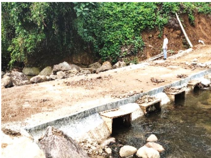
Build river crossing
