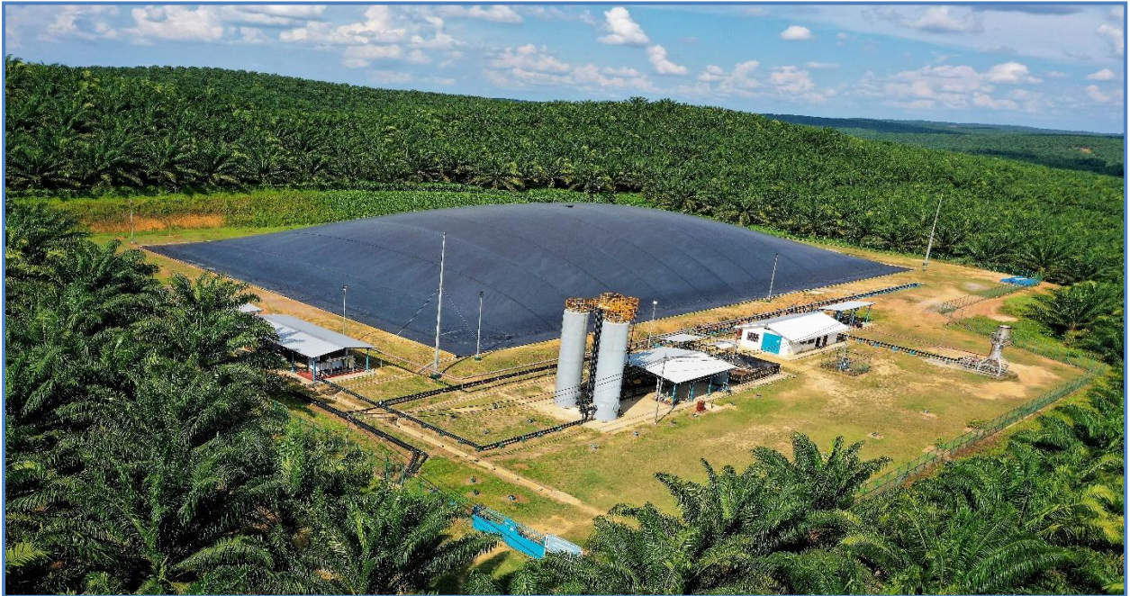
Biogas plant in North Sumatera
