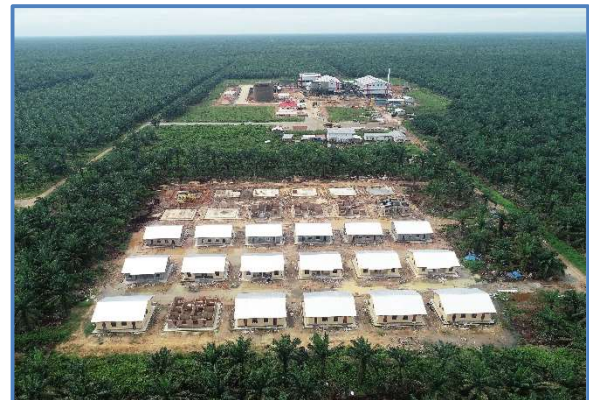
Construction of new employees' housing
