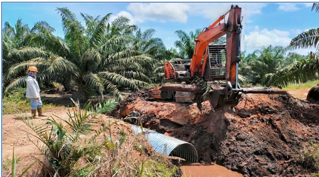
Steel culvert replaced to improve drainage
