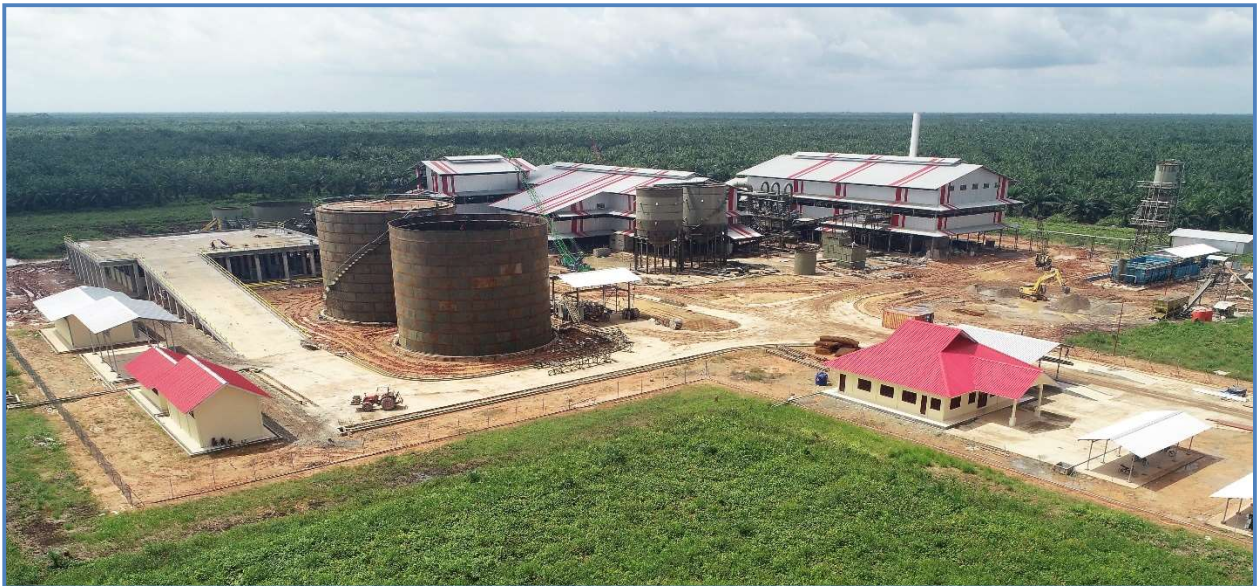
HPP mill in North Sumatera taking shape
