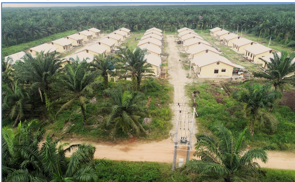
Electrification of workers housing in HPP
