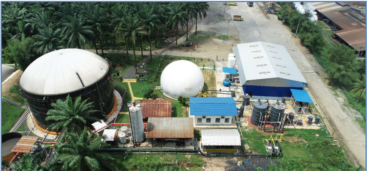
Newly built BioCNG Plant in Blankahan
