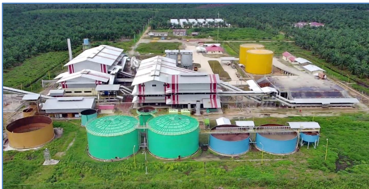
HPP Mill finally completed
