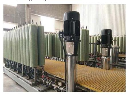
(2) Treatment of 50 tons of leachate per day at a landfill in Heilongjiang Province, China. In processing leachate, DTRO filtration has the advantages of high stability for long periods of time, high and stable water recovery, less clogging of membranes, stain resistance and low contamination qualities and a long lifespan. The overall recovery rate for the wastewater at this facility is approximately 75%.
