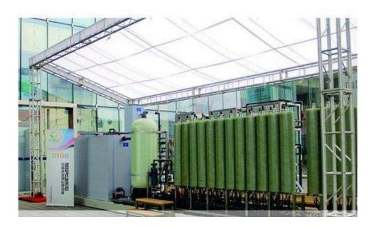
(3) Treatment of desulfurized wastewater and reuse at a power plant located in Harbin City, China. Desulfurized wastewater from power plants normally comes with the problems of hard water, muddy and high salinity. DTRO technology was used to resolve these issues and reuse the wastewater at this electric power plant and achieved near zero emissions. The overall recovery rate for recycled wastewater at this plant is approximately 75%.
