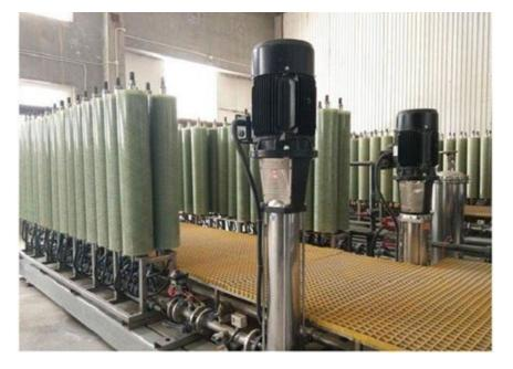
(2) Treatment of leachate (1,000 tons per day) at a garbage landfill site in Shaanxi Province, China. In processing landfill leachate, DTRO technology, compared with traditional technologies, has the advantages of higher operation stability, consistent high water recovery rate, more fouling-resistant, and a longer lifespan.
