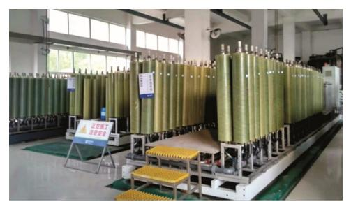
(3) Zero Liquid Discharge (ZLD) project at a power plant located in Shandong, China. Due to the severe air pollution problems in China, the Chinese government has imposed stringent regulations on power plant air and liquid emission. DTRO filtration was used as the essential component in the wastewater treatment system to filter wastewater and ultimately achieve ZLD.
