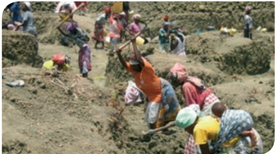
Community members digging the dam by hand.
