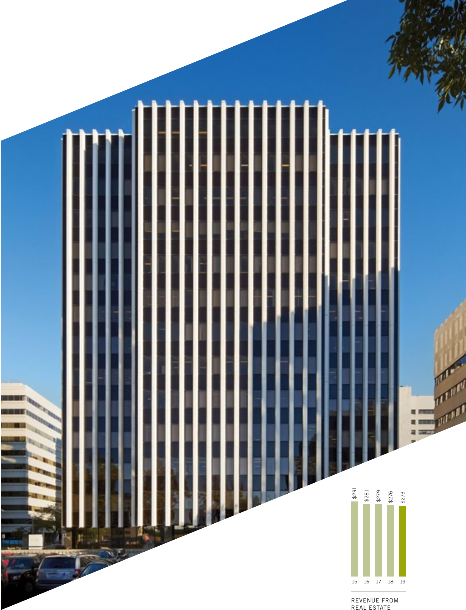
Petroleum Plaza, Edmonton, AB
