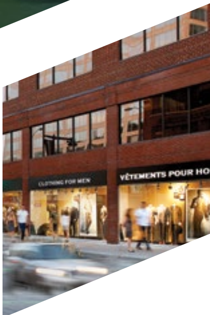
301 Laurier Avenue, Ottawa, ON
