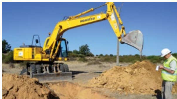
Geotechnical test pitting in the area of the Project water dams
