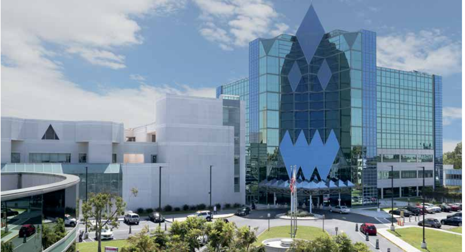
St. Francis Medical Center Lynwood, California
