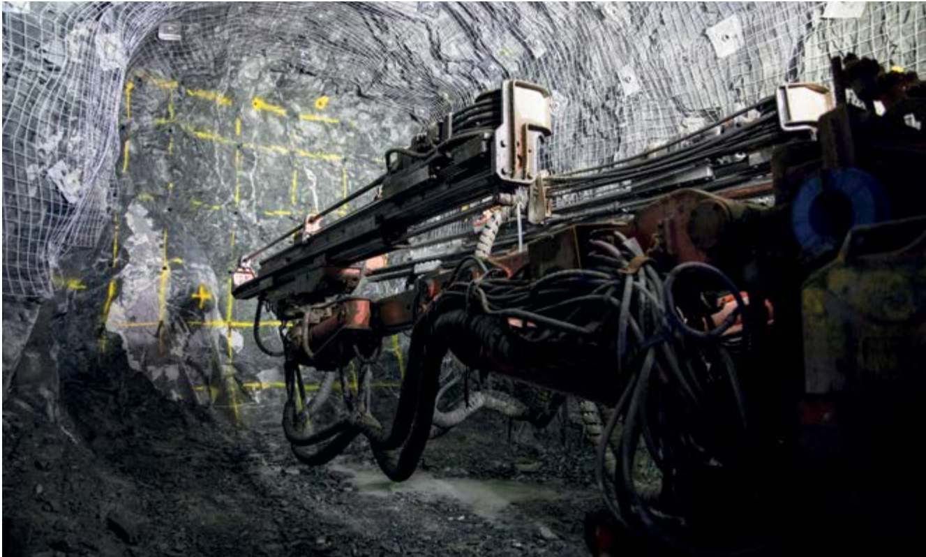
Underground mining at Jaguar
