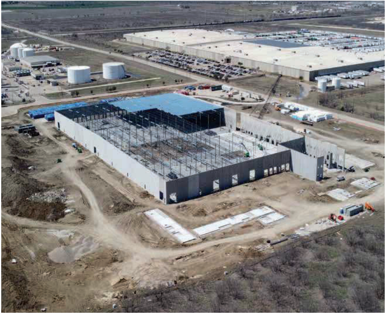
Mega facility under construction in Midlothian, Texas
