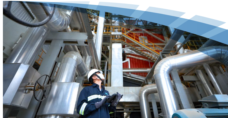
Two biomass generators at our plant in Bangkok, Thailand (shown here) have reduced our consumption of natural gas resulting in the reduction of 40,000 MTCO 2e from our greenhouse gas (GHG) inventory.
