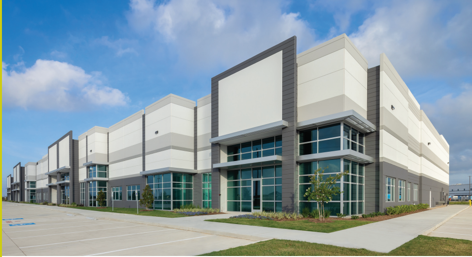
Grand West Crossing, Houston, Texas
