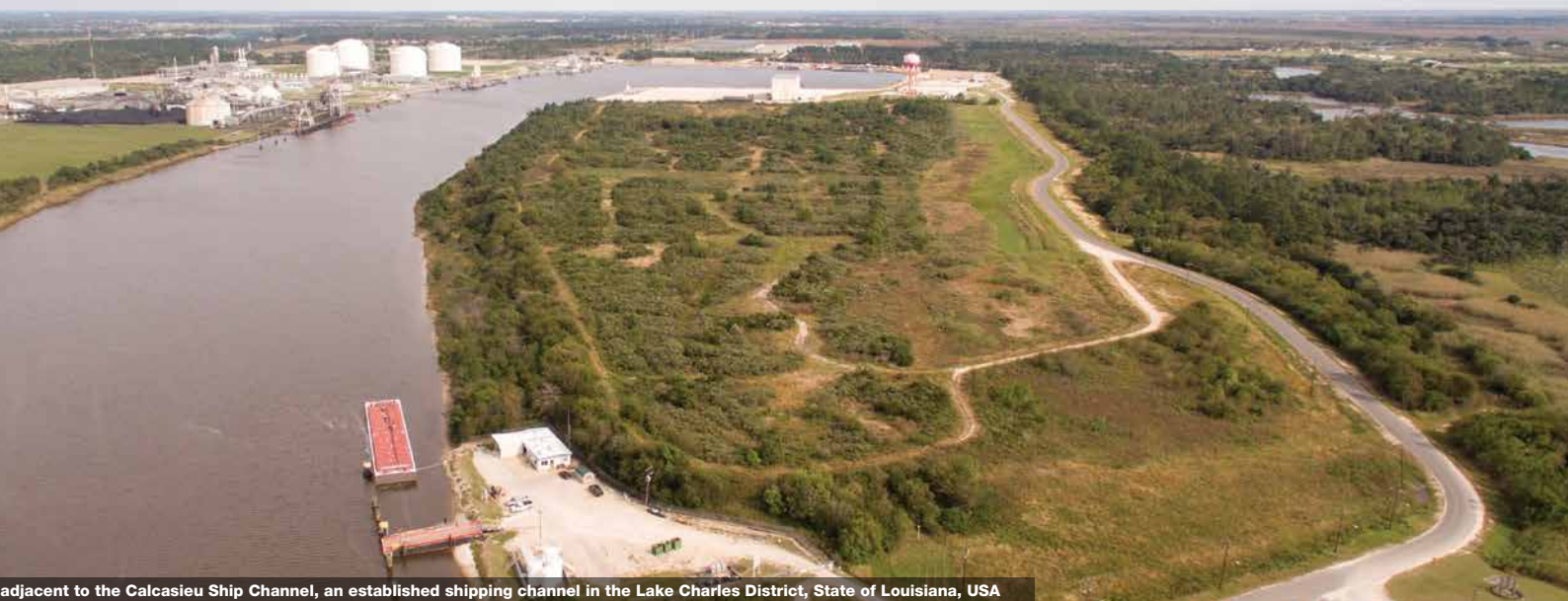
adjacent to the Calcasieu Ship Channel, an established shipping channel in the Lake Charles District, State of Louisiana, USA
