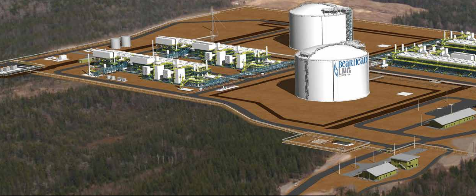
Artist's rendition of the 8 – 12 mtpa (design capacity) Bear Head LNG project at Point Tupper, Richmond County, Nova Scotia, Canada
