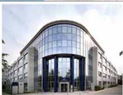
LEOPOLDSTRASSE 252, 252A AND 252B | $33.9 M
