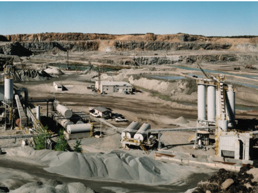
Tilcon New York's Mount Hope facility in Wharton, New Jersey is one of the largest granite quarries in the US. Mount Hope operates 24 hours a day with a 2,300 tph crushing plant, three on-site asphalt plants and a soil remediation plant. Acquired in April 2001, the facility is centrally located to serve the densely populated and heavily travelled northern New Jersey and New York City markets.
