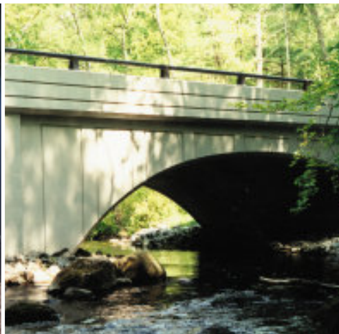
Below: This precast concrete arch bridge from Oldcastle Precast’s Rehoboth facility allowed fast-track construction while preserving the tranquillity of Buck Horn’s Brook in rustic Rhode Island, USA.
