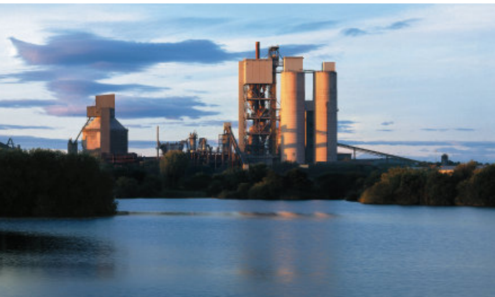
Situated on the river Shannon close to Limerick City, Irish Cement operates a modern one million tonnes capacity cement plant.
