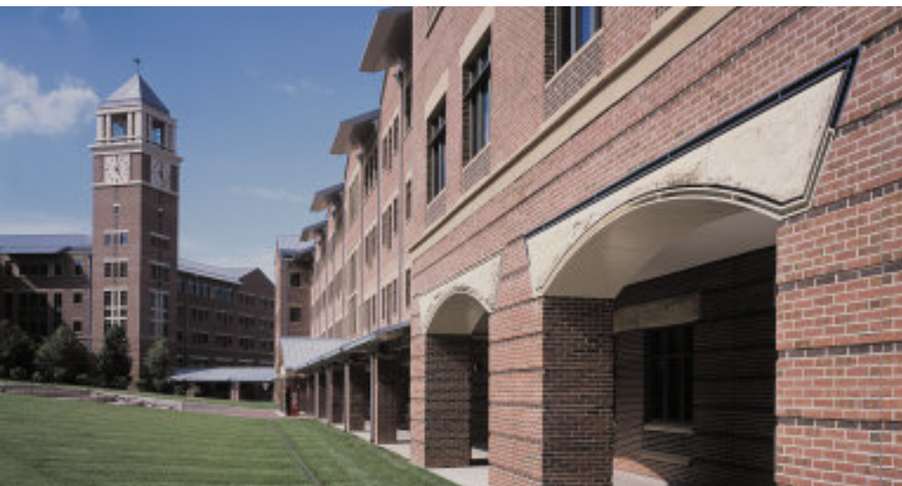
Sprint's 200-acre World HQ campus in Kansas City incorporated 7.5 million facing bricks from three different Glen-Gery plants.
