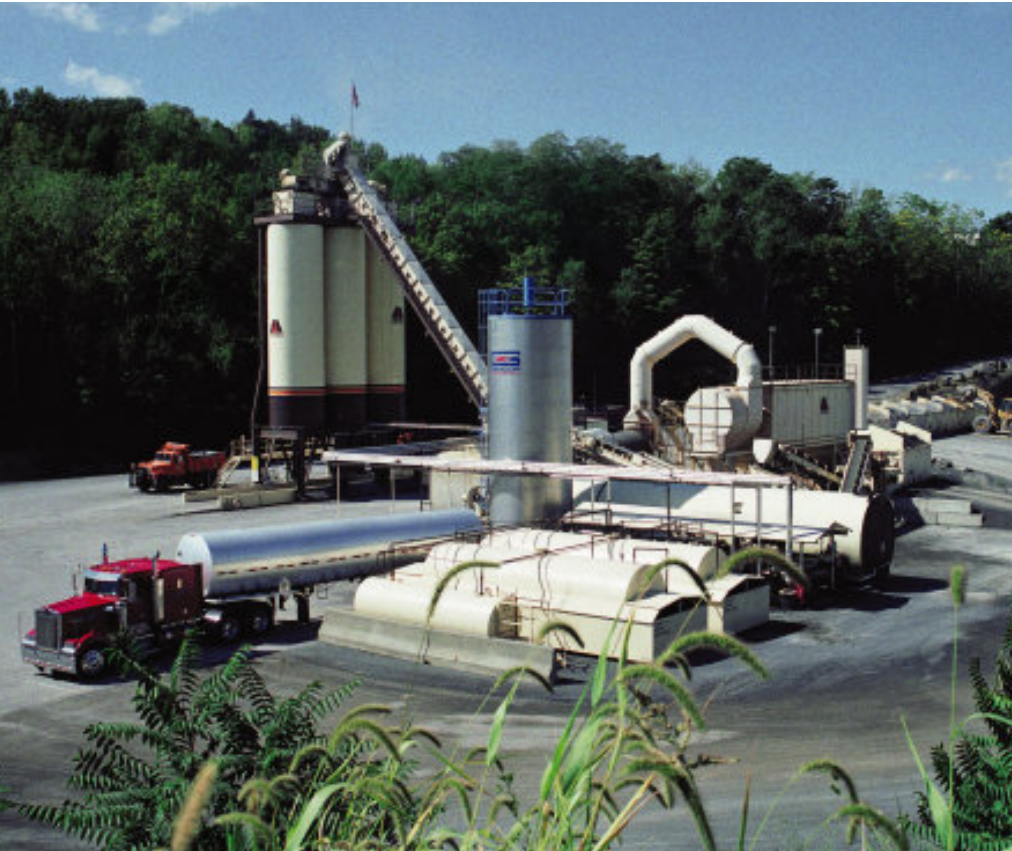
A recipient of the National Asphalt Pavement Association's Diamond Achievement Award, this 350 tph Callanan plant is a major producer of recycled asphalt mixes at East Kingston, NY.
