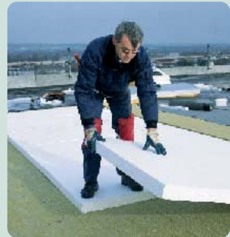
Above: ThermiSol EPS being applied to a roof in Denmark.
