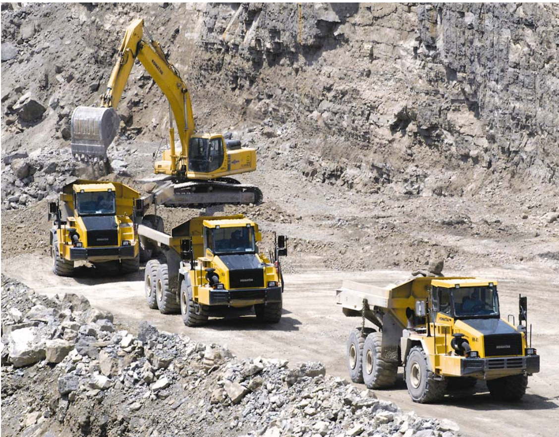
Workers at The Shelly Company's Marble Cliff Quarry in Hilliard, Ohio remove shot rock in preparation for expanding the mine to include an underground operation. A US$12 million capital expenditure project, the underground mine will allow Shelly to retrieve 90 million tonnes of high-quality friction-grade material while continuing its surface mine operation that produces non-friction commercial-grade material. The mine is scheduled to go underground in early-2006.
