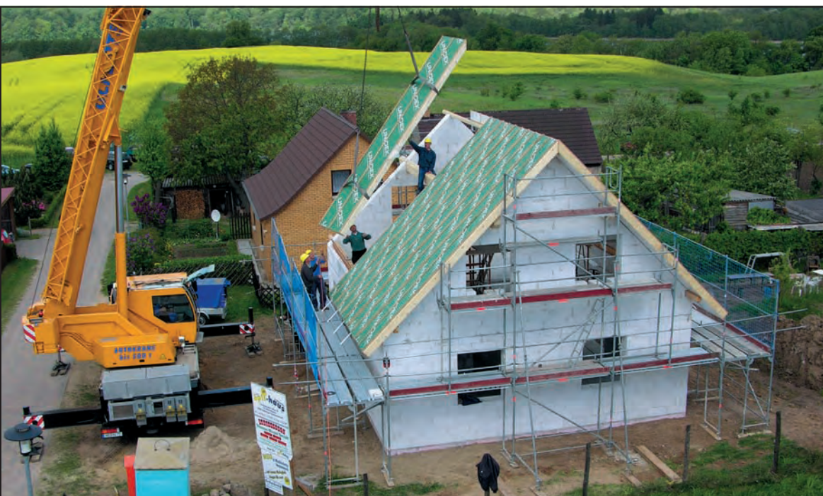
Uni-Plan Plus self-supporting insulation sandwich roofing elements are manufactured in the Netherlands by Unidek. Fitted on roof beams, these innovative elements remove the need for the traditional roof tile support system used in conventional pitched building construction, reducing building time with considerable savings on building costs.
