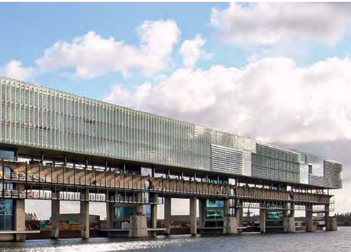
Brakel Atmos developed the innovative movable Glastec façades as well as the glass roof structure of the 548-metre Kraanspoor building in Amsterdam harbour. This project received the Glas Award 2008 and the MIPIM Award.
