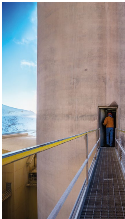
A Production Supervisor enters the homogenising silos at Ash Grove's Plant in Durkee, Oregon. The Durkee Plant produces more than 1m tonnes of clinker annually and employs approximately 120 people. Production at the plant began in 1979.
