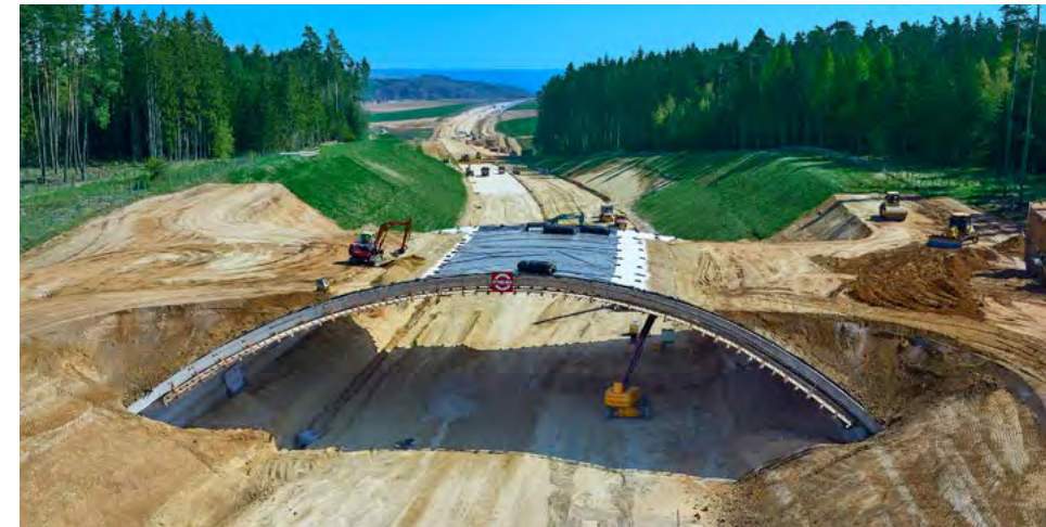
OPTERRA, part of CRH's Europe Materials Division, supplied concrete for this 'green bridge' on the Bundesstraße motorway project in Southern Bavaria, Germany. The project, which runs through a forest area, includes a new motorway as well as 14 additional structures. The green bridge, completed in May 2019, will enable wildlife to cross the busy motorway, thus reducing the impact of the project on the area's biodiversity.
