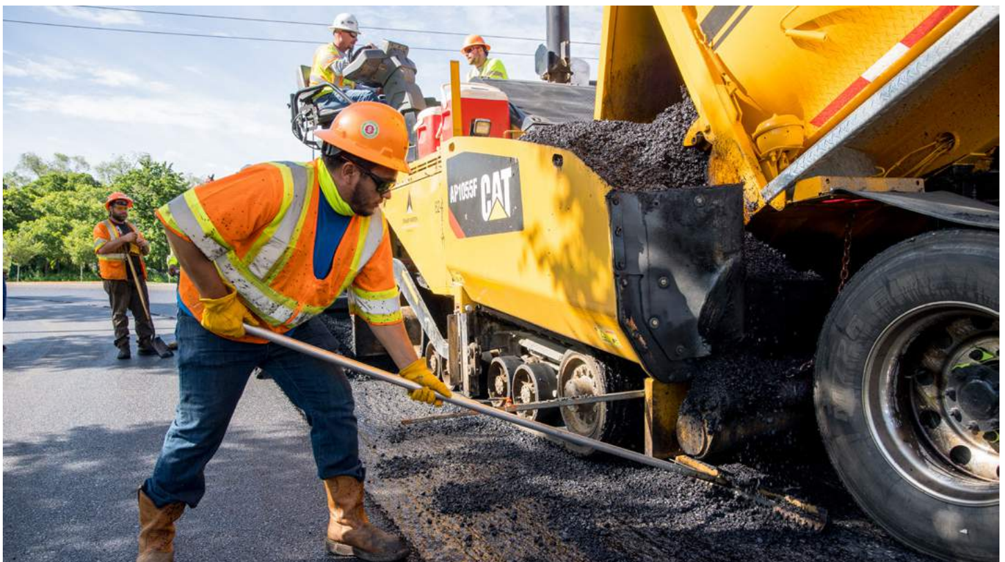
Staker Parson Materials & Construction, part of CRH's Americas Materials Division is a leading provider of paving, concrete, construction services and landscaping in Utah. CRH is the largest producer of asphalt in North America. The material is 100% recyclable which helps make CRH a significant contributor to the circular economy.
