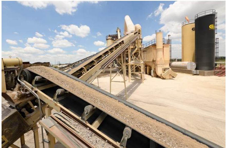
An asphalt plant at Alvarado, Texas. CRH is the largest producer of asphalt in North America. As a 100% recyclable product it helps to make CRH a significant contributor to the circular economy.
