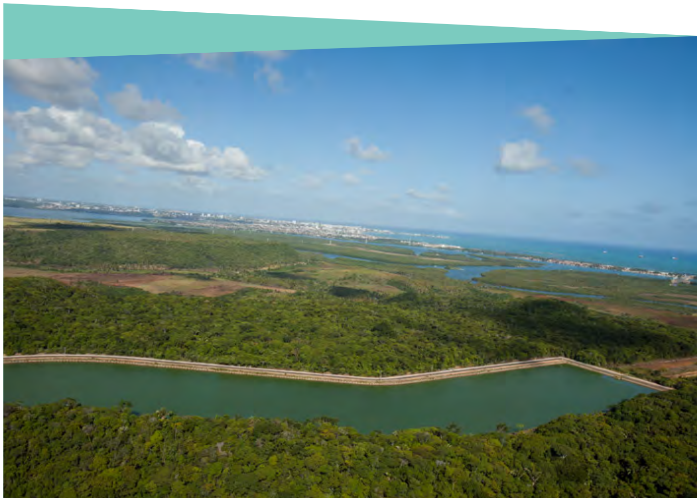
Wastewater treatment plant at the PVC unit in Maceió (AL)
