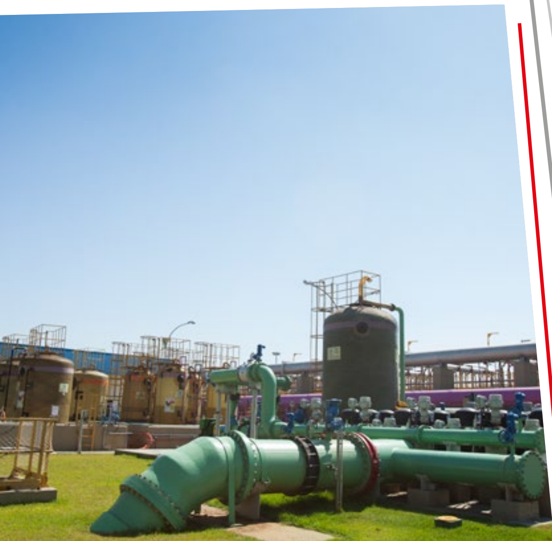
Water treatment plant in Santo André (SP)
