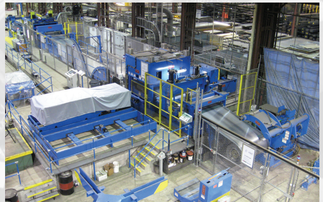
Modernization Stretcher Levellers - Winnipeg North & B&T Steel Cut-To-Length Line - Arrow Steel
