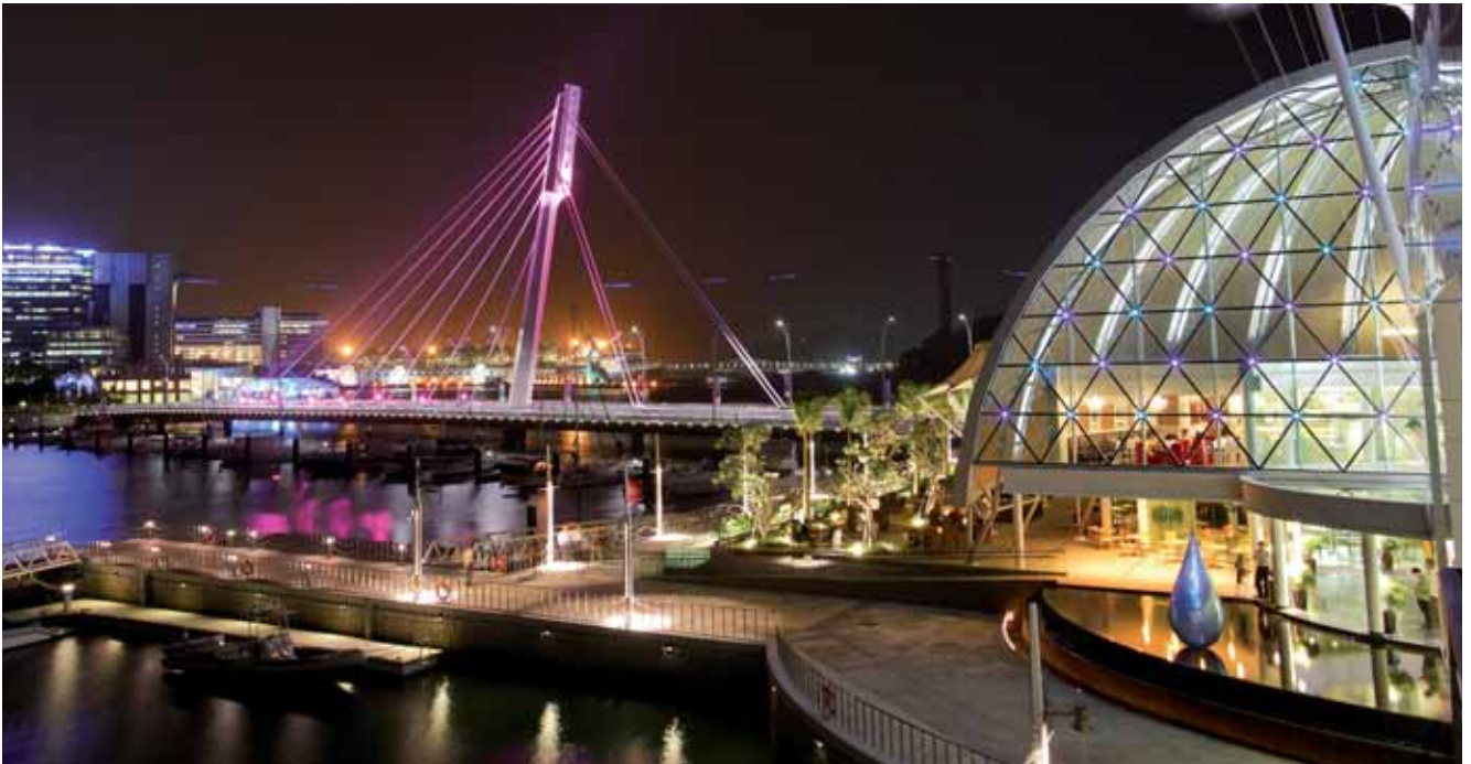
Keppel Bay Bridge is part of the masterplan and infrastructure in the transformation of Keppel Bay into a premier waterfront precinct.
